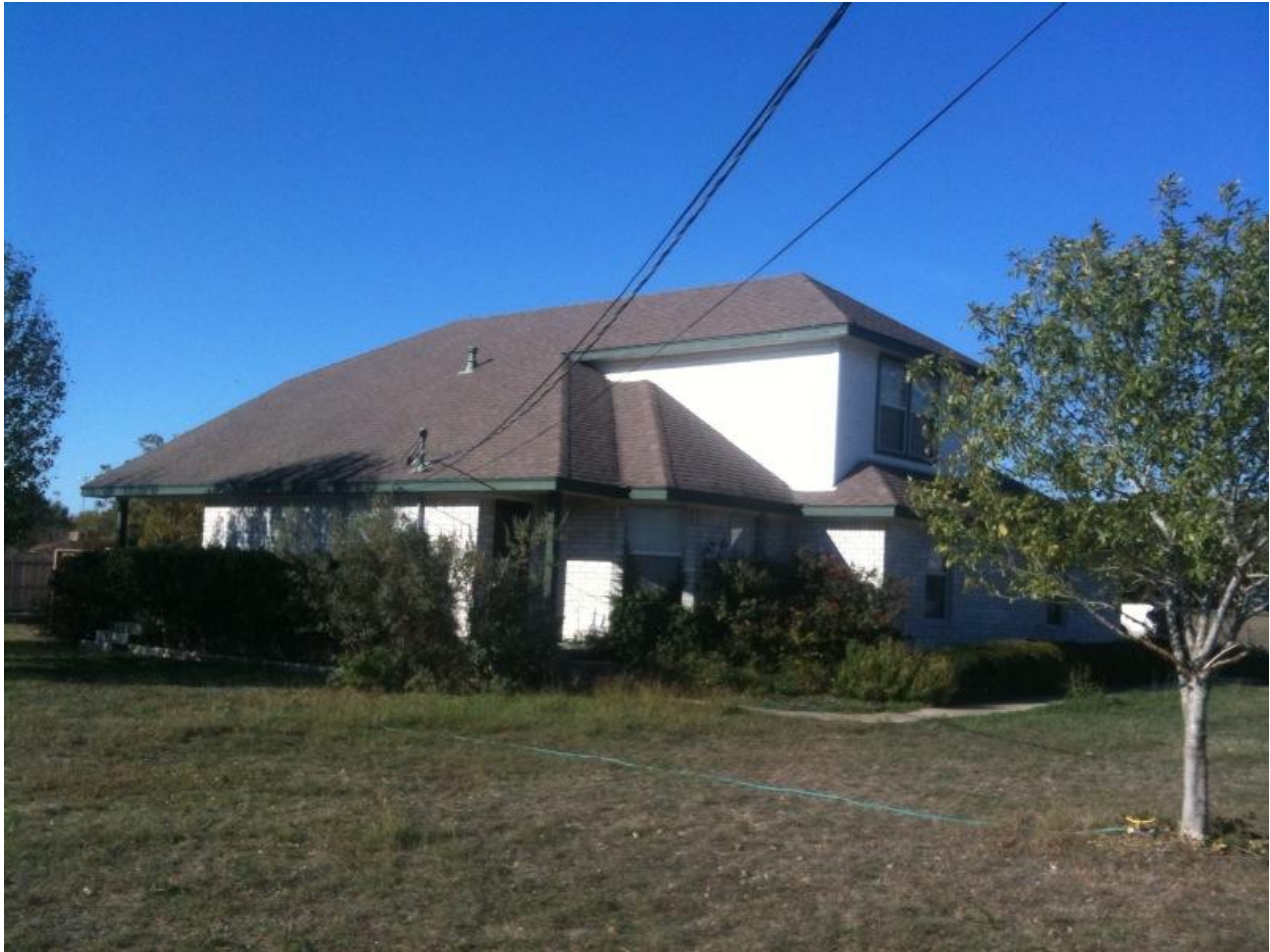
Figure F-2 Photo of Mountain City City Hall Building
