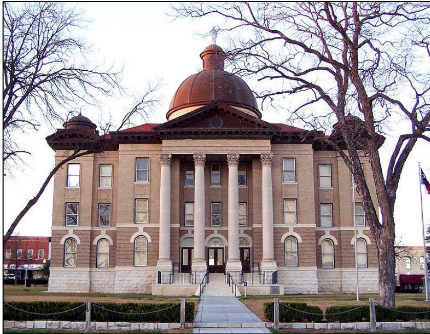
Figure 6 Hays County Courthouse (Source: Wikipedia – Hays County)
