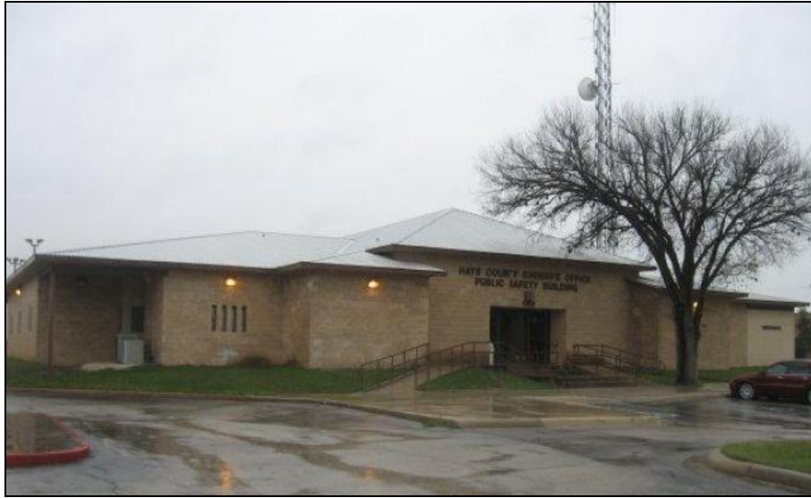
Figure 35 Hays County Public Safety Building (Source: Property Appraisal Report Hays County, 2010)
