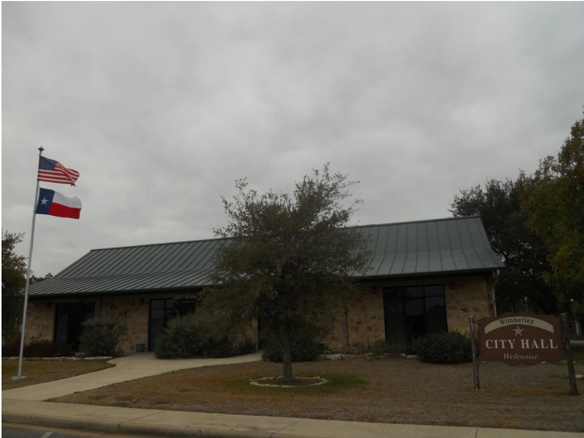
Figure J-2 Wimberley City Hall (Source: Wimberley)
