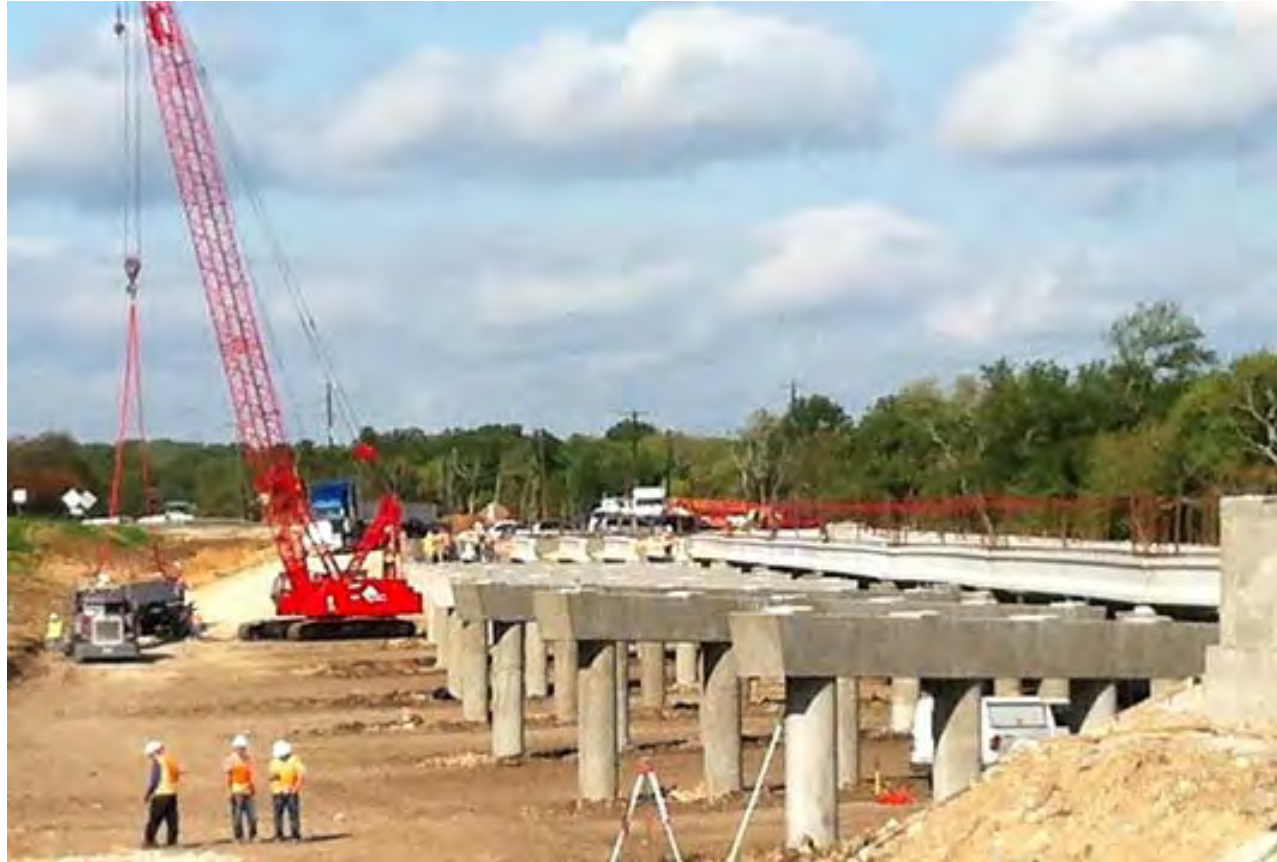
Setting bridge beams
