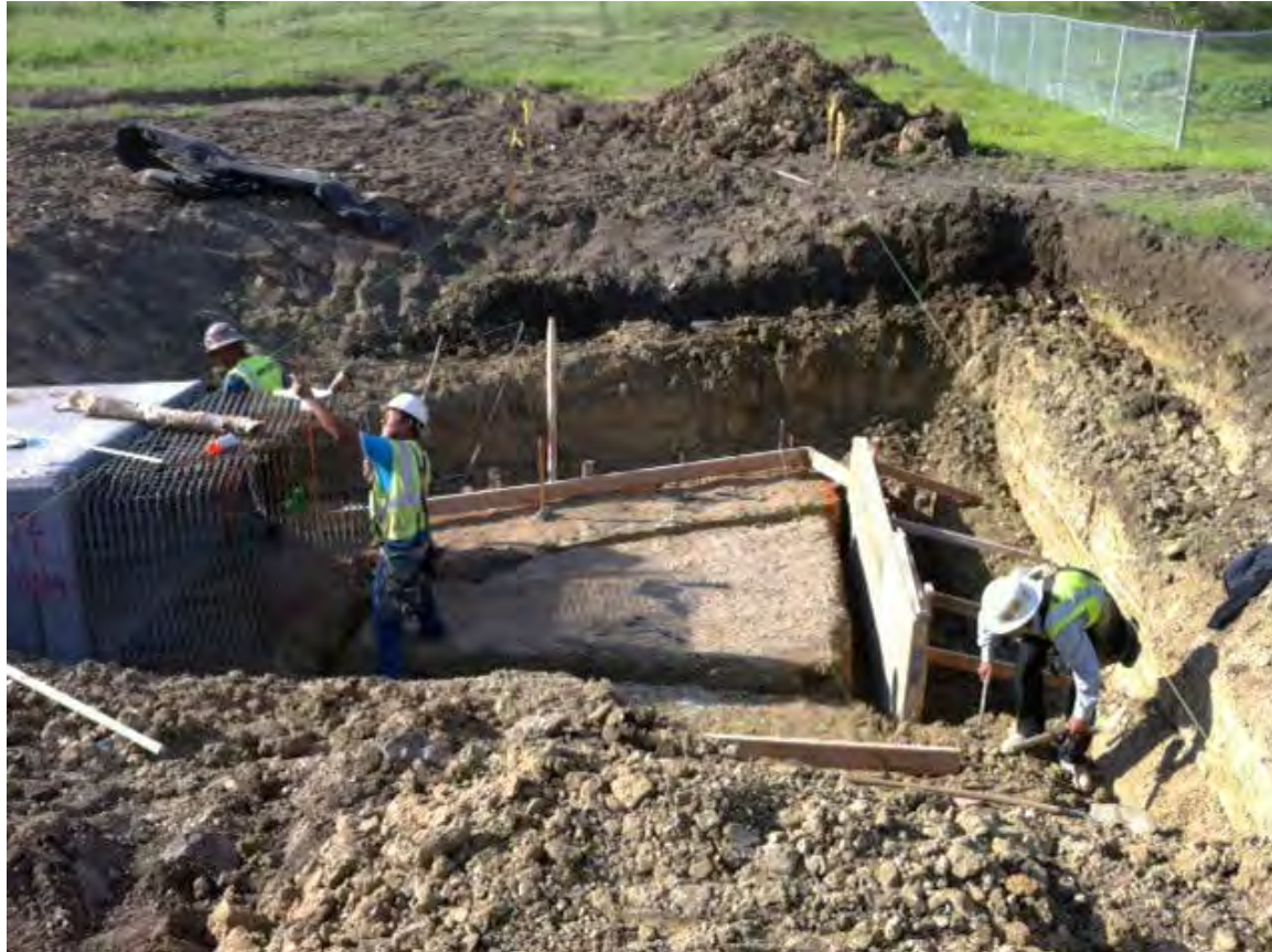
Forming extension and apron of Culvert B
