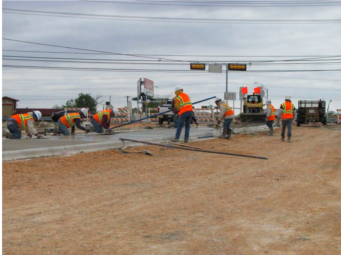
Finishing newly poured concrete median
