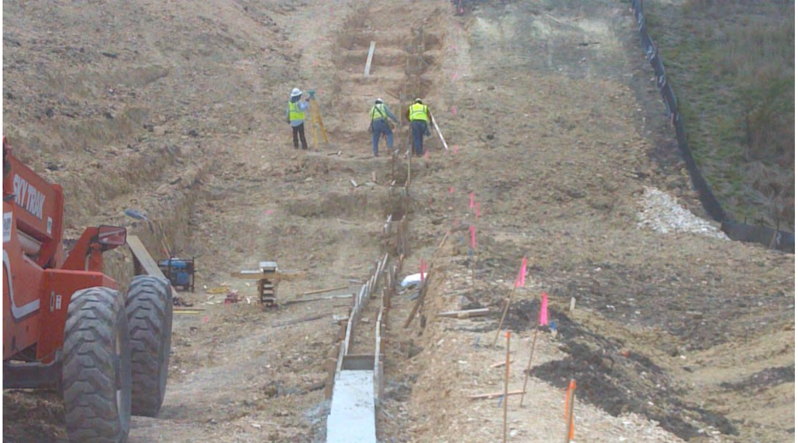
Forming leveling pad for MSE Wall
