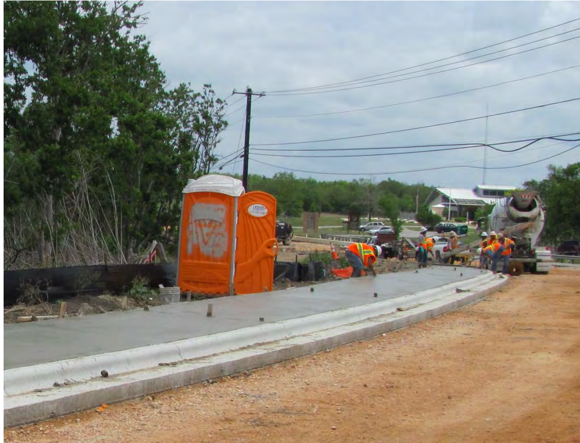
Pouring and finishing concrete sidewalk
