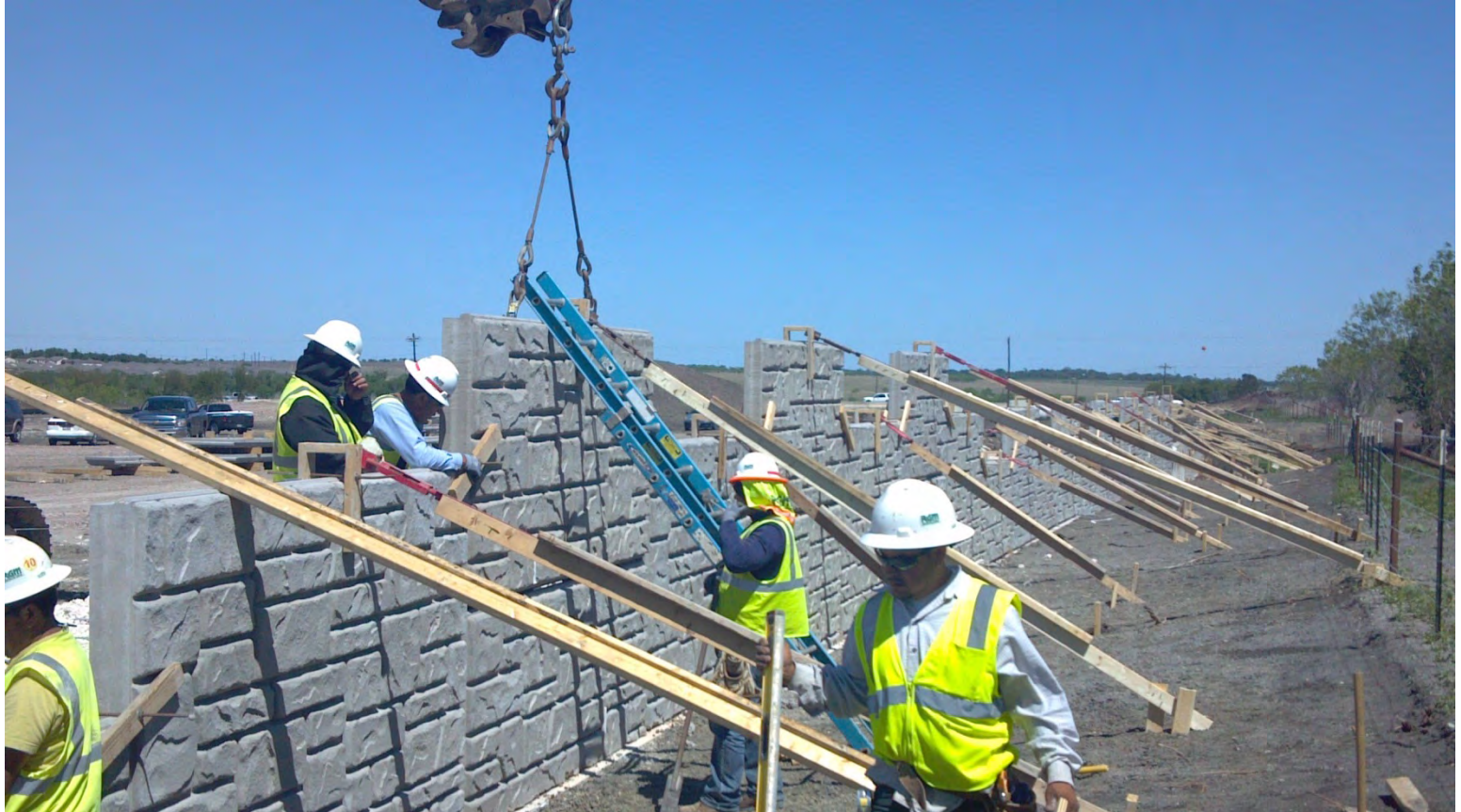
Placing MSW Wall panels and bracing
